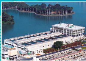
澄清水湖高級淨水處理設備工程 Chenchin Lake Advanced Water Treatment Plant
