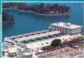
龍潭湖高級淨水處理設備工程 Chendun Lake Advanced Water Treatment Plant
